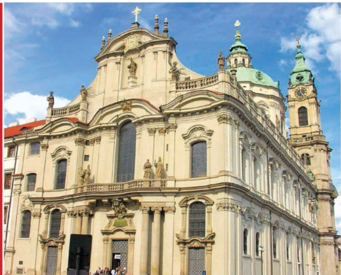
(This and above) The Church of St. Nicholas
